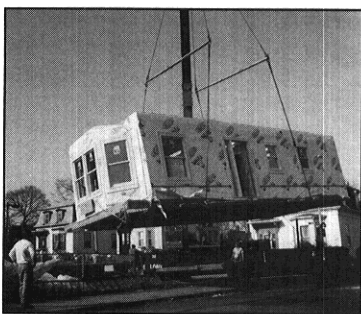
Dorchester Bay Buildable Lots (during construction).
