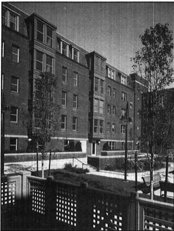
Langham Court (completed).
