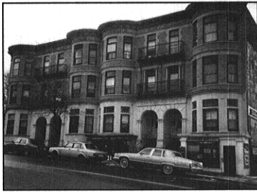
Humboldt Avenue Apartments (pre-construction).
